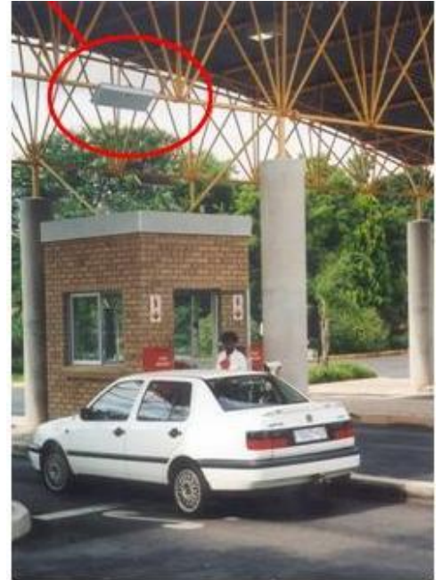
RFID controlled entrance – Reader circled.
